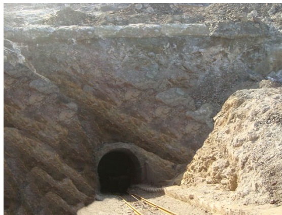
Fig. 1 The environment of the Adit
