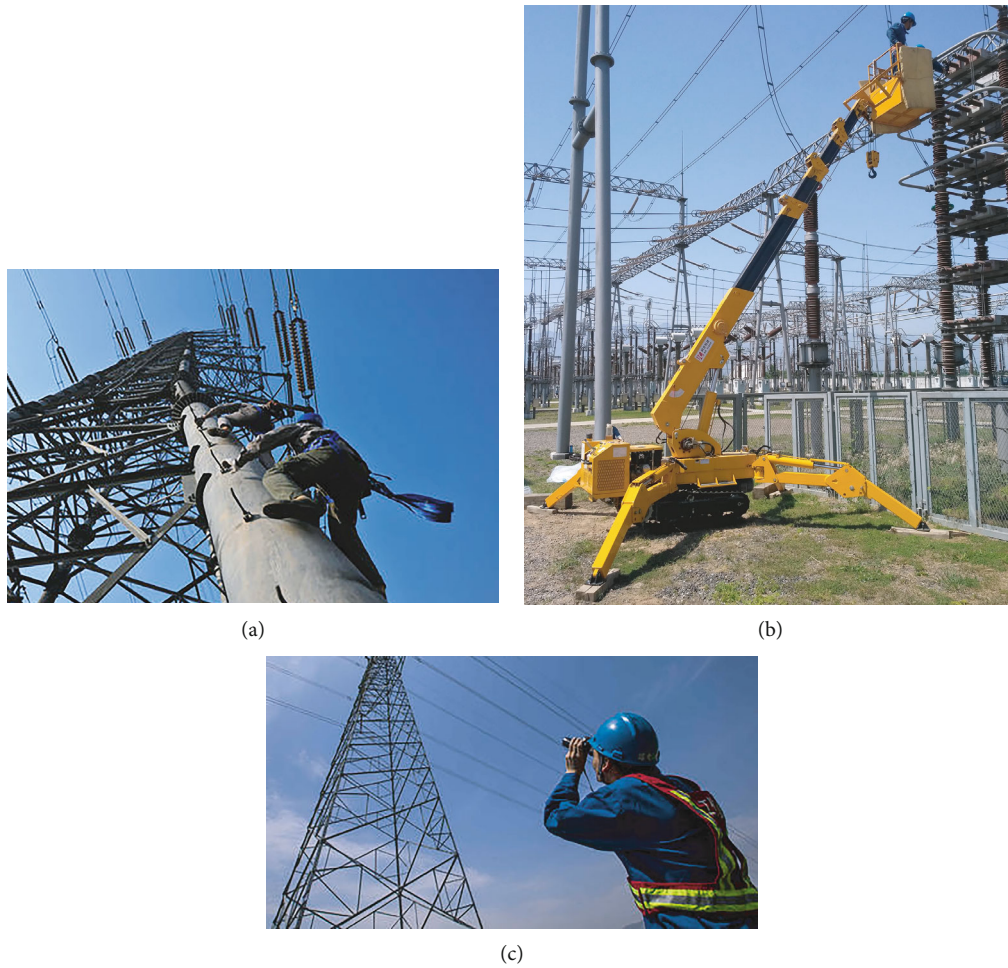
FIGURE 1: Traditional inspection methods: (a) line crawling inspection; (b) ground-based inspection; (c) manual inspection with a telescope.
